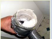
moved to clean the combustible lint from under it and to clean and check the connector (left) for holes and/or deterioration, and to determine if the connector is of the proper type.
